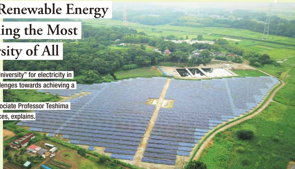
Noda Mega Solar Power Plant—the largest solar power plant owned by a university in Japan
